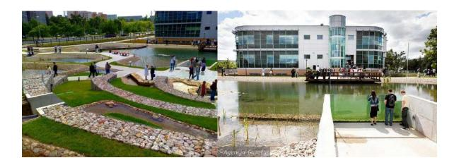
2. Rain water reservoir, filtering green roofs and filtration system in Kłobucka street. A housing development with about 3000 m<sup>2</sup> water surface, (30 min stay), 35 min travel time.
